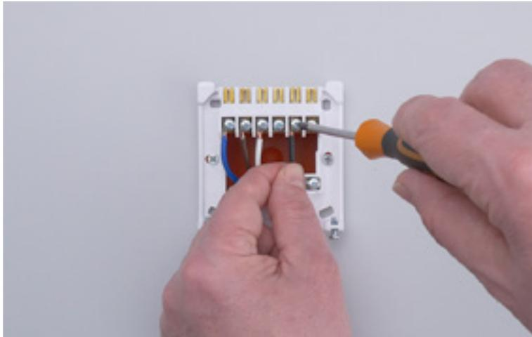
Connect the wires to their corresponding terminals on the new backplate:
